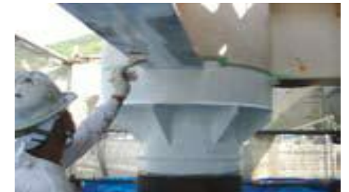
Titanium foil corrosion prevention system
